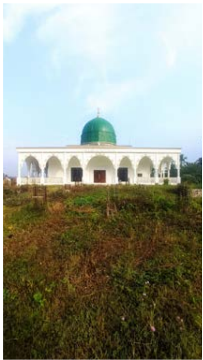
Construction of Boys Campus Mosque
