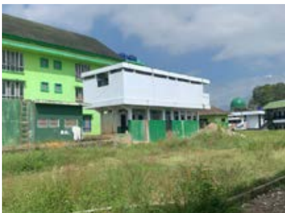
Construction of 2nd Floor for toilet, its behind the Indonesia Building
