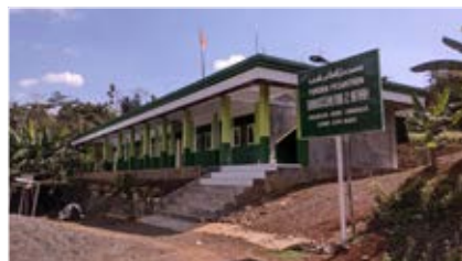
Construction of 5 Local Classrooms at Darussalam 2 Afiah
