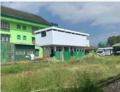
Construction of 2nd Floor for toilet, its behind the Indonesia Building
