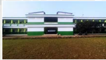
Construction of Sewindu Building 2nd Floor and Stairs
