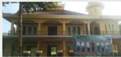
Ummahatul Mu'minin Mosque Renovation
