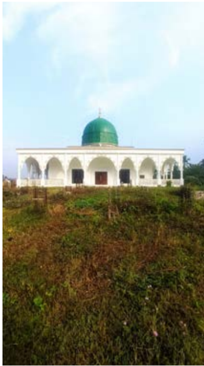
Construction of Boys Campus Mosque
